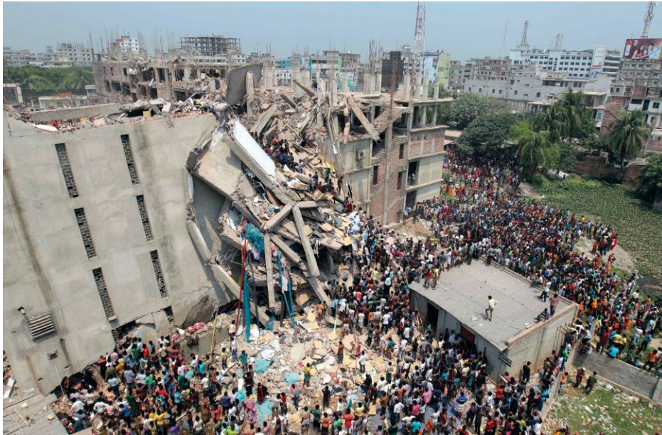
More than 1,120 people, mostly garment workers, were killed in April 2013, after the Rana Plaza building in Bangladesh collapsed.
